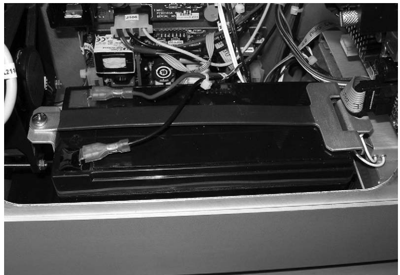
Figure 4-26 Battery removal BAT2100A
